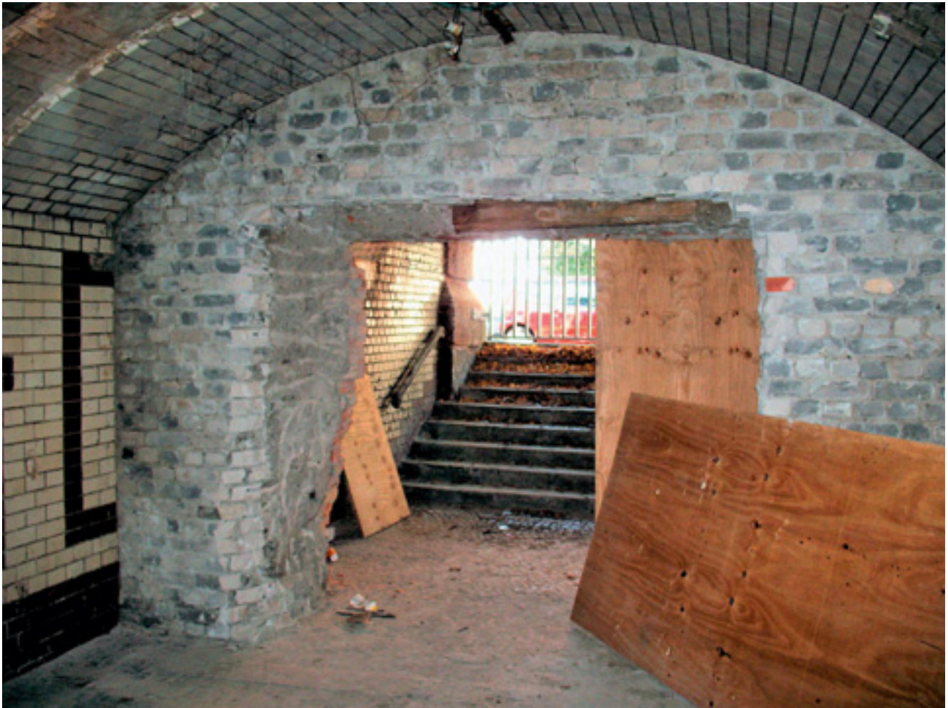
Stettiner Tunnel (Foto: wikipedia / Franz Richter BY-SA 3.0)
